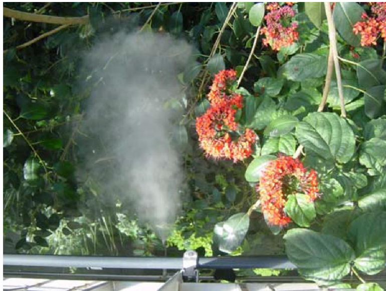
Fog nozzle delivering a small-droplet mist for evaporative cooling
